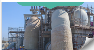
MANIFOLD REPLACEMENT PROJECT
